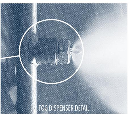
The follies are constructed from lightweight, recycled high density plastic, which has a hollow core containing the water distribution system for the fog dispensers. The piping system is linked to a series of fog dispenser nozzles, integrated at regular intervals into the folly frame structure. The fog dispensers are high pressure valves which release water vapour, as a result of high pressure water within the piping system.
